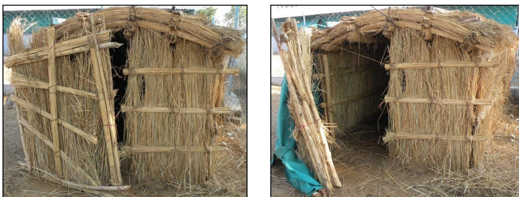
Fig 29. Low cost Hut- type shed for cold protection
